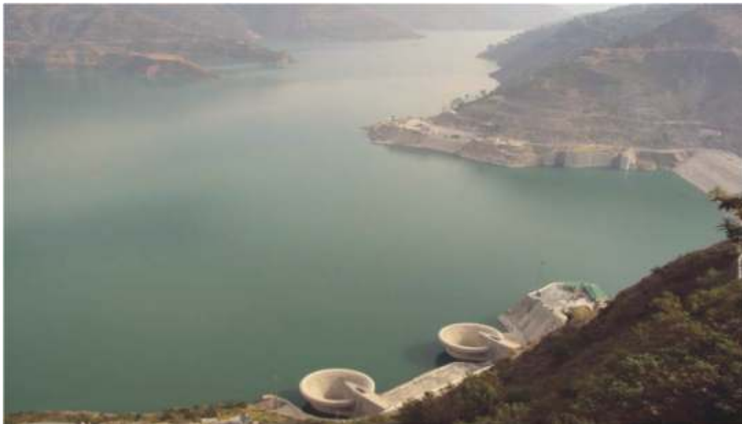
A view of Right Bank Shaft Spillway of Tehri Dam Site
